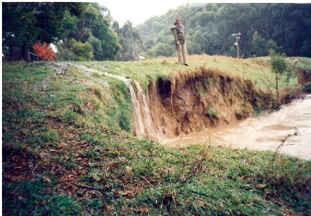
Figure 31: Stream bank erosion on the Stockyard Creek
