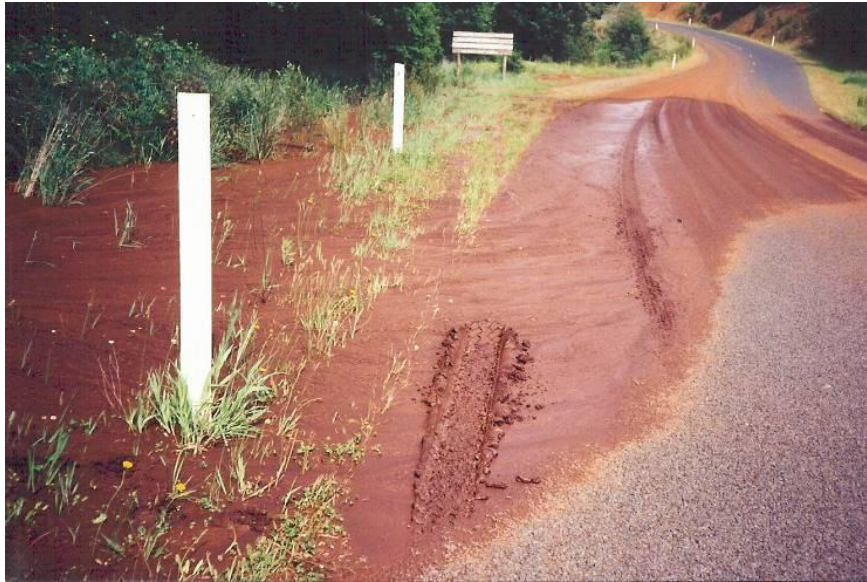
Figure 6: Sediment covering the road surface is an example of an off-site impact of soil erosion
