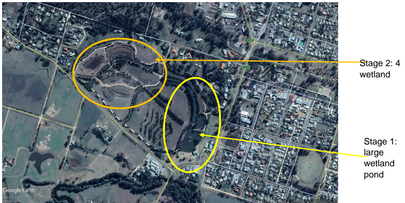
Figure 1: Aerial Photograph of Heyfield Wetlands. Stage 2 ponds.
