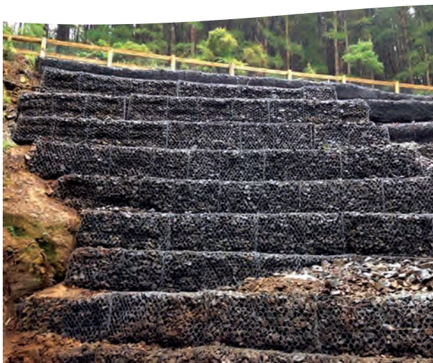
Pictured: works on waterways completed at Turton's Creek in South Gippsland
