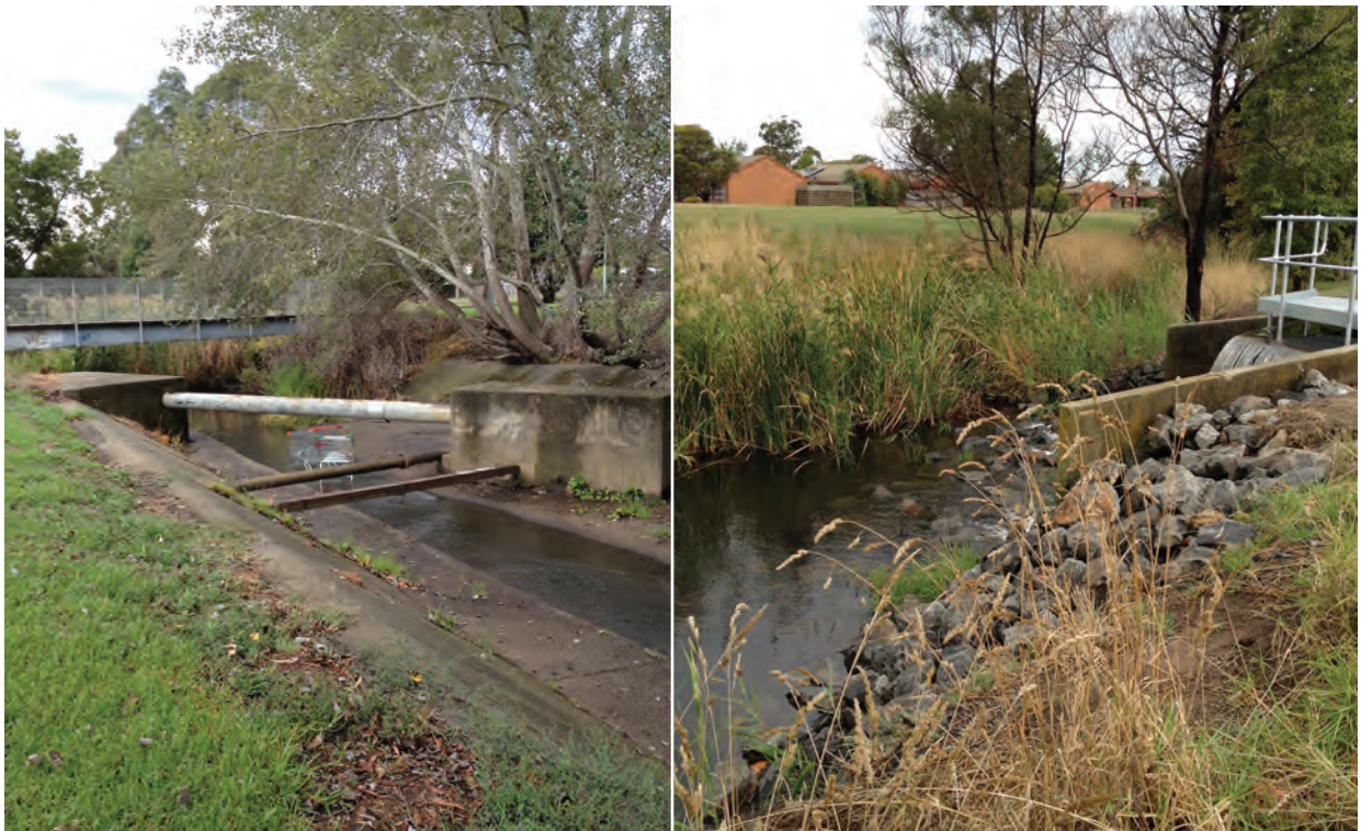
Figure 14 – Township reach showing lack of overhanging native vegetation, channelisation and concrete lining of the stream channel and the outlet from Lake Kernot
