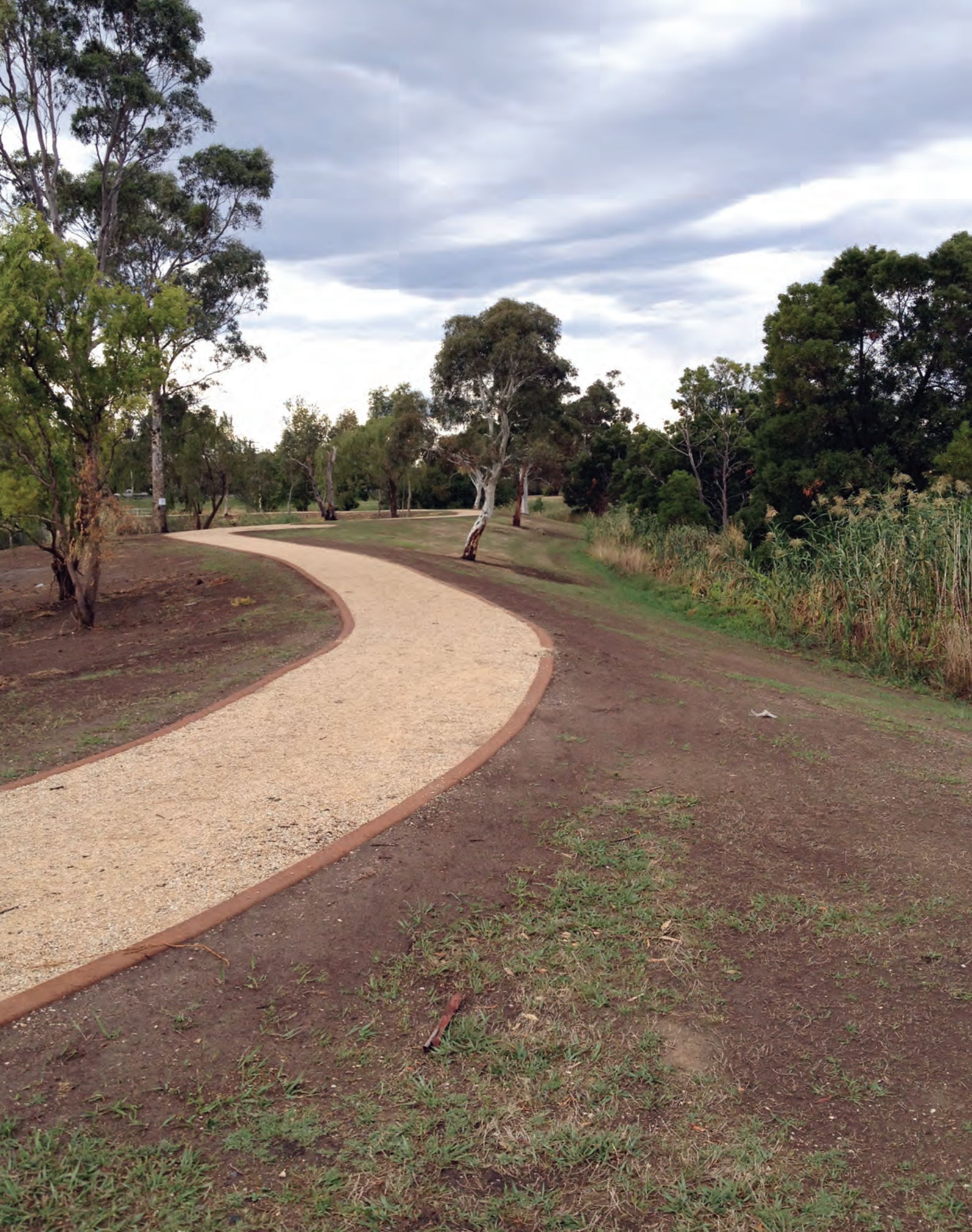
Reach 3a (Township Reach) – Lake Kernot pathway running alongside Waterhole Creek
