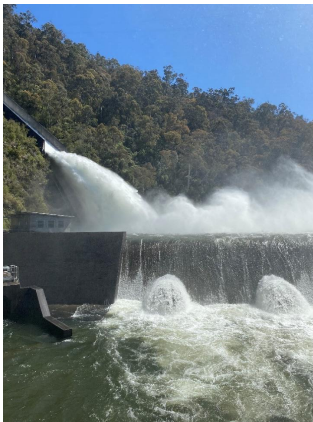
Figure 16 Thomson River - active spillway in November 2022
