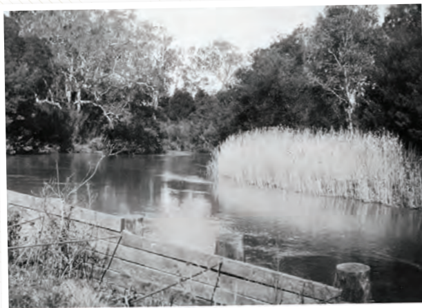
Bellbird Corner at the Bellbird corner bridge, circa 1930s. Photo courtesy Duncan Fraser
