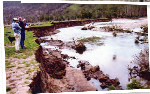
Inspecting the damage at Licola after 2007 floods
