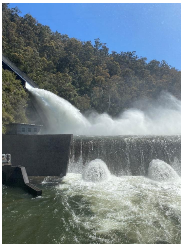
Figure 16 Thomson River - active spillway in November 2022
