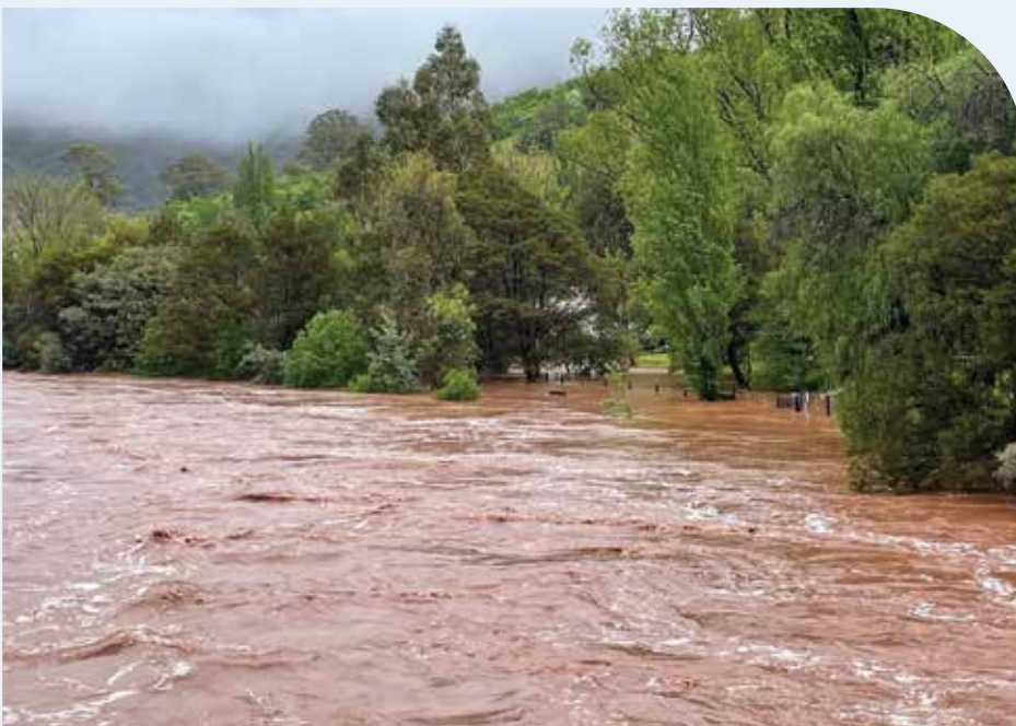
Floods at Licola on the Wirn wirndook Yeerung (Macalister River) October 2023. Image West Gippsland CMA.
