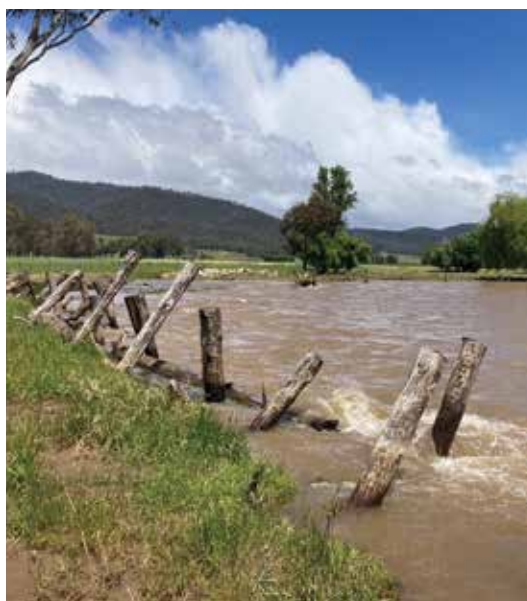
Above: Timber revetment on Corryong Creek during flooding in late 2022. Image North East CMA.
