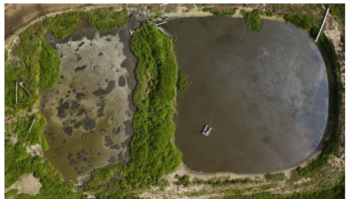
Figure 1, Steve and Jess' two pond effluent system, linked to their pipe and riser infrastructure.
