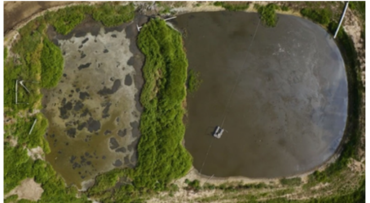
Steve and Jess's two-pond effluent system
