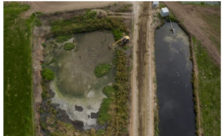
Tom's two-pond effluent system
