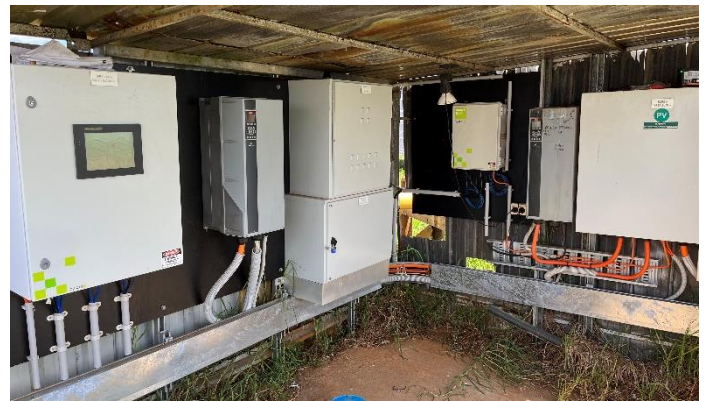
Figure 4, Wilandra's AEI SmartBox system paired with an AEI irrigation control box and variable speed drives for both bore and irrigation pumps.
