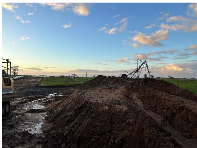
Figure 13: Pivot tipped over and severely damaged 17-03-23
