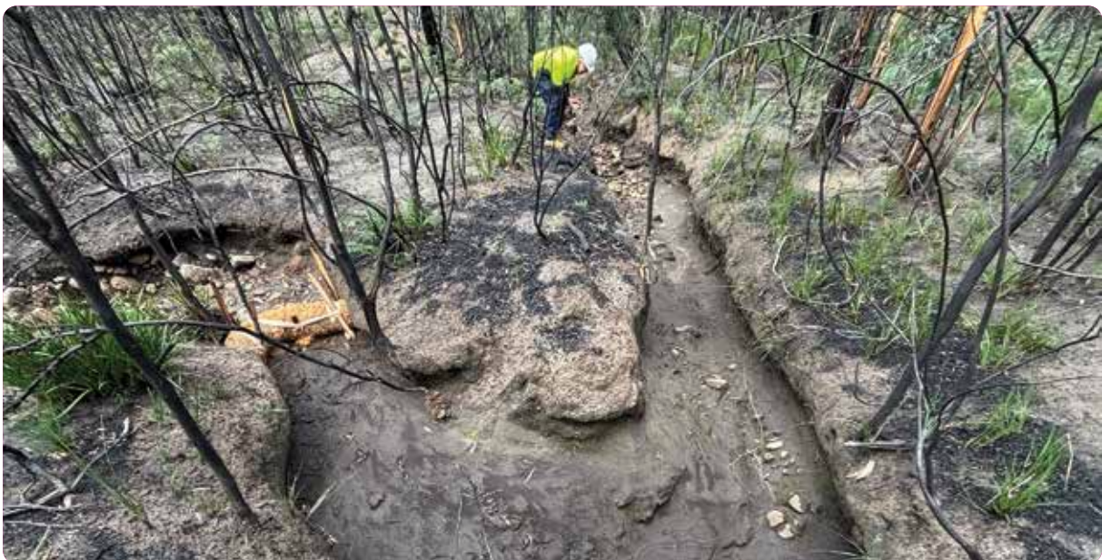
The Grampians (Gariwerd) were impacted by bushfires in late 2024 and 2025 and repair work has now begun through Glenelg Hopkins CMA funded works to support waterway resilience post fire.
