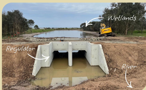
Heart Morass regulator under construction
